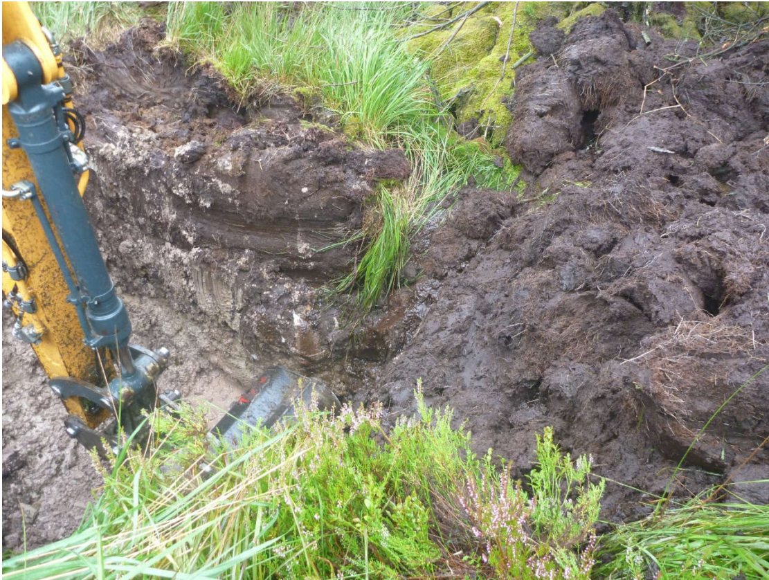
Trial Pit T4 – Photo 3
