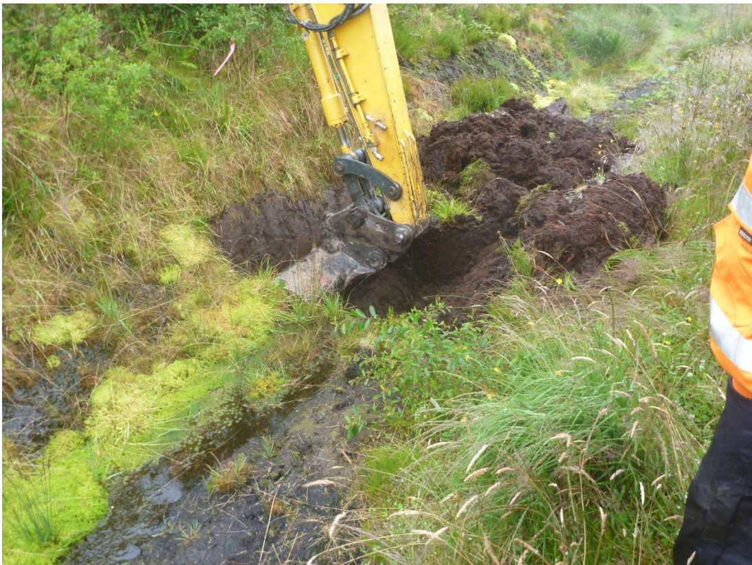
Trial Pit T19 – Photo 2
