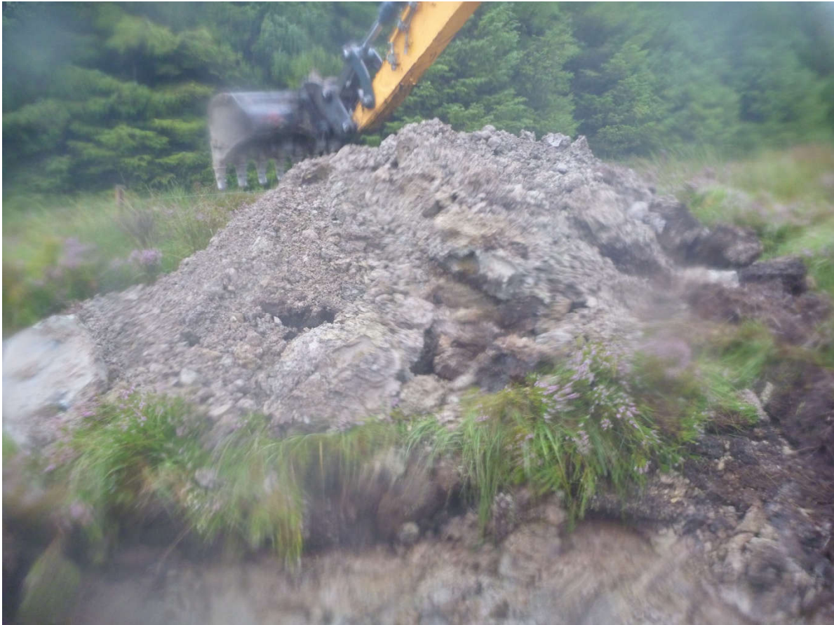
Trial Pit T8 – Photo 1
