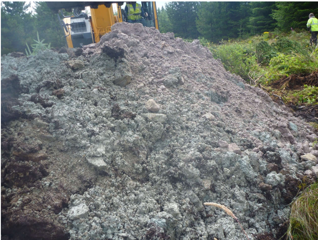
Trial Pit T6 – Photo 2
