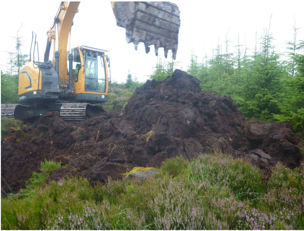
Trial Pit T18 – Photo 3
