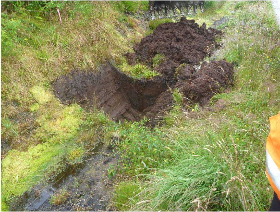
Trial Pit T19 – Photo 3
