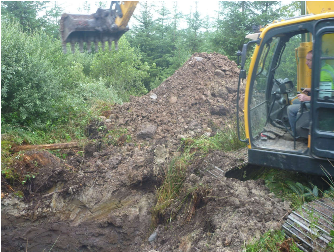
Trial Pit T11 – Photo 4
