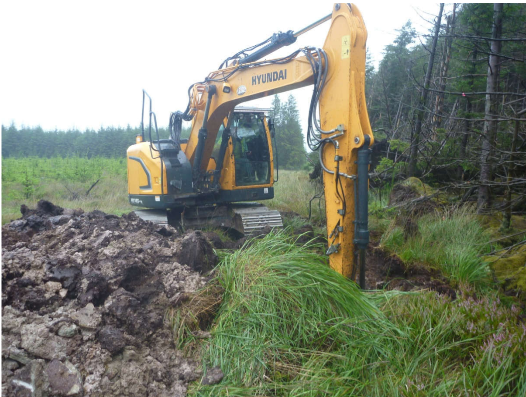
Trial Pit T4 – Photo 2
