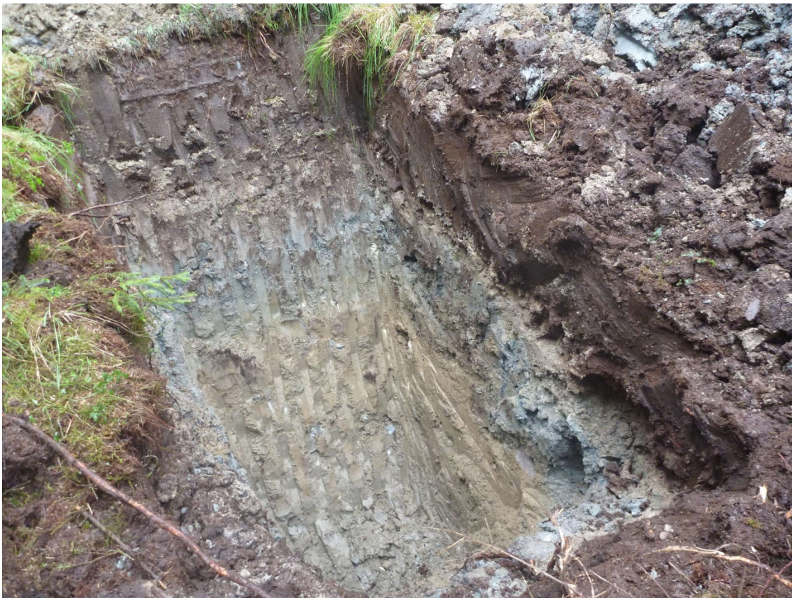
Trial Pit T10 – Photo 4
